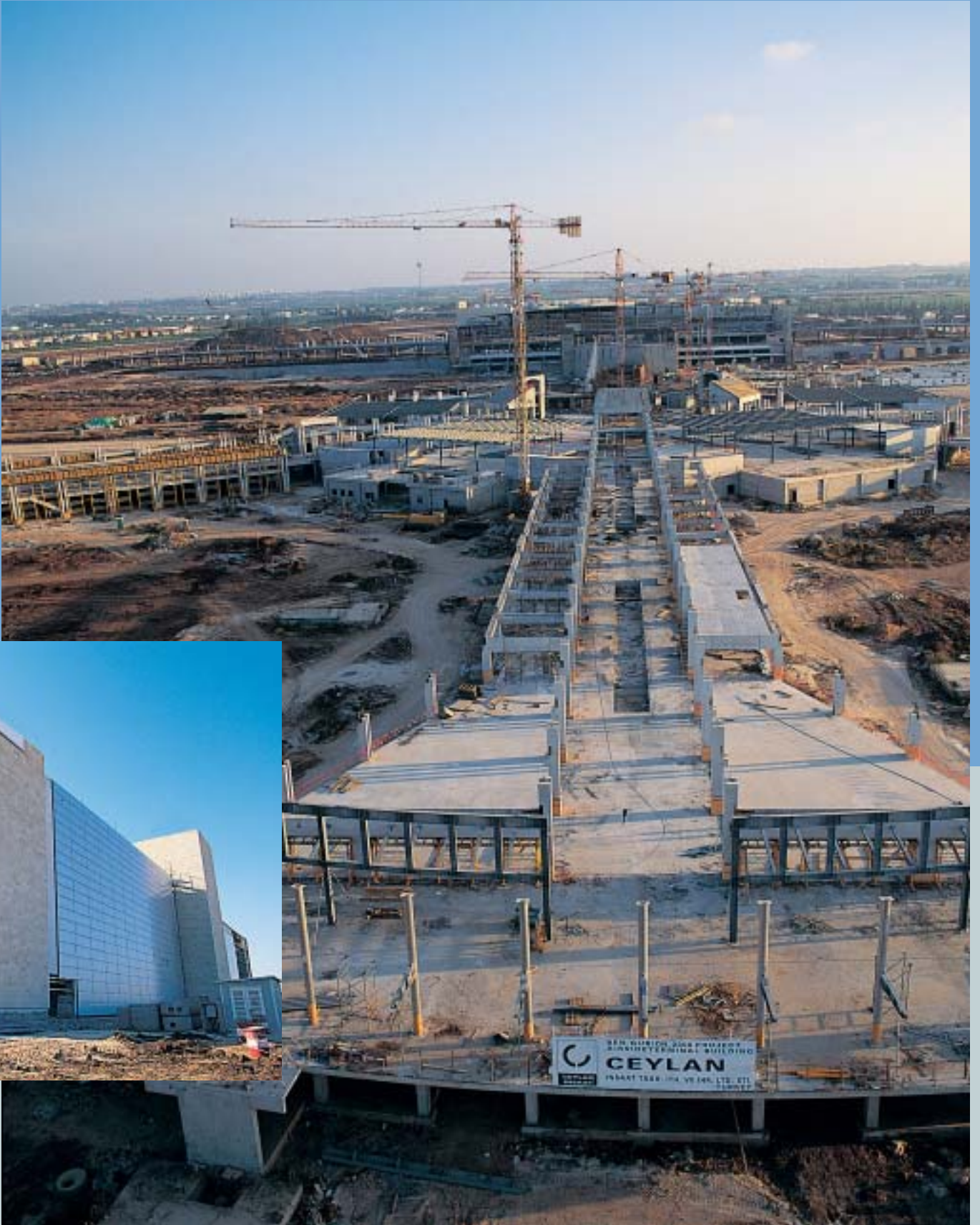
▶ The Rotunda, 160 m in diameter, covers an area of 20,000 sq m; three concourses connect to 24 aircraft through airbridges.
